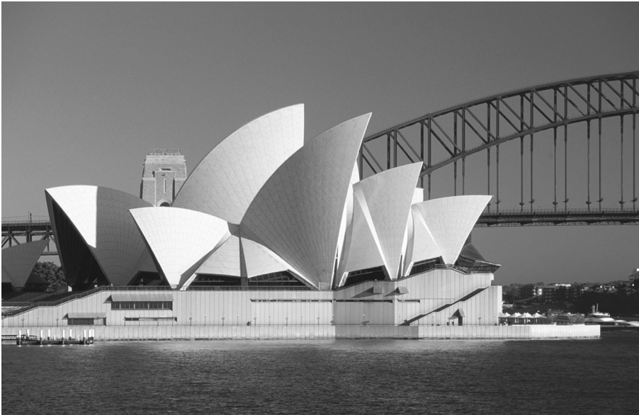
Figure 1 Sydney Opera House was envisaged as a sculptural element in a magnificent harbour setting. It consists of a substantial, solid platform that draws on historic references. Atop the platform are the shells, constructed as segmented precast concrete ribs, overlaid with glittering white glazed tiles. (Courtesy Max Dupain & Associates)
